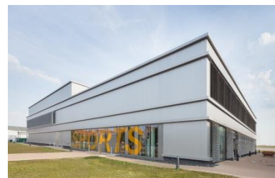
Physical Fitness Center, Katterbach
