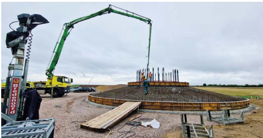
Windparkbau in Gau-Bickelheim.
